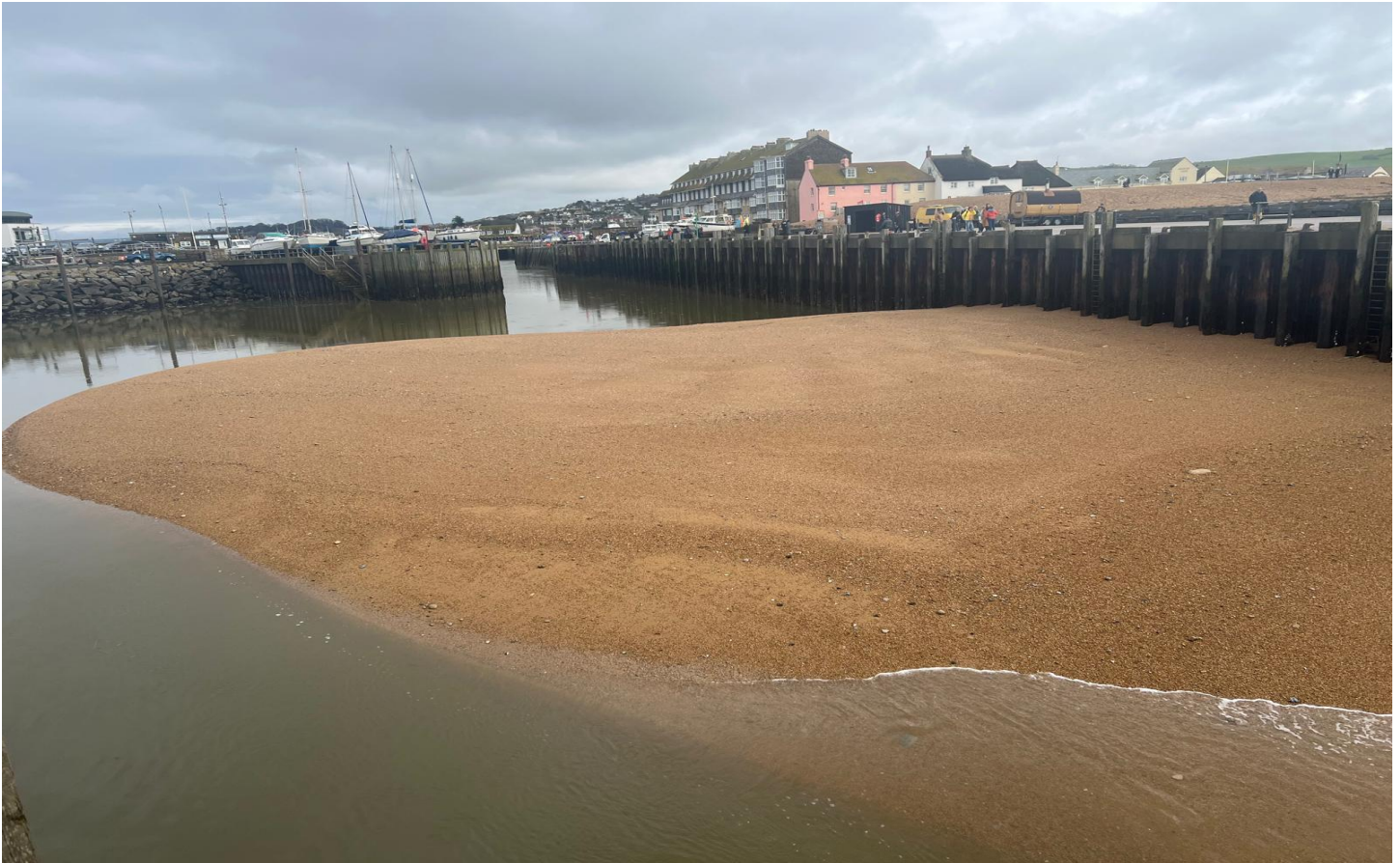
The next photo shows how far the beach has migrated seaward, now extending approximately 40–50 metres further out than before the storms. The beach line has advanced beyond the end of the rock groyne, clearly illustrating the scale of movement.
